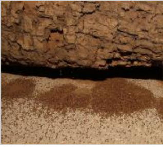
Death watch beetle damage and frass
